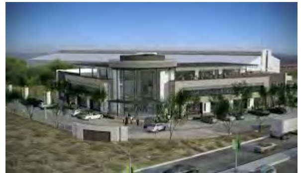
Rehabilitated Wetland Clairwood Logistics Park with acknowledgement to Rising Sun
